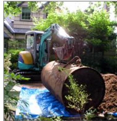
*Removal of an underground tank* more commonly, completely filling the clean tank with a DEQ-approved material, such as sand or concrete slurry. Voluntary decommissioning certification, per Oregon DEQ, requires soil samples with acceptable concentrations of petroleum.
